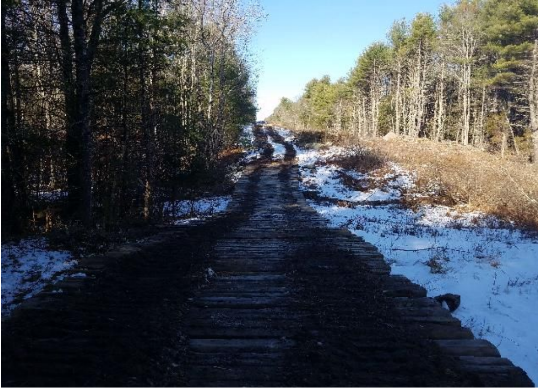
Fig 3: Building access road from Str 85 to 83. Viewing west. (03-26-20).
