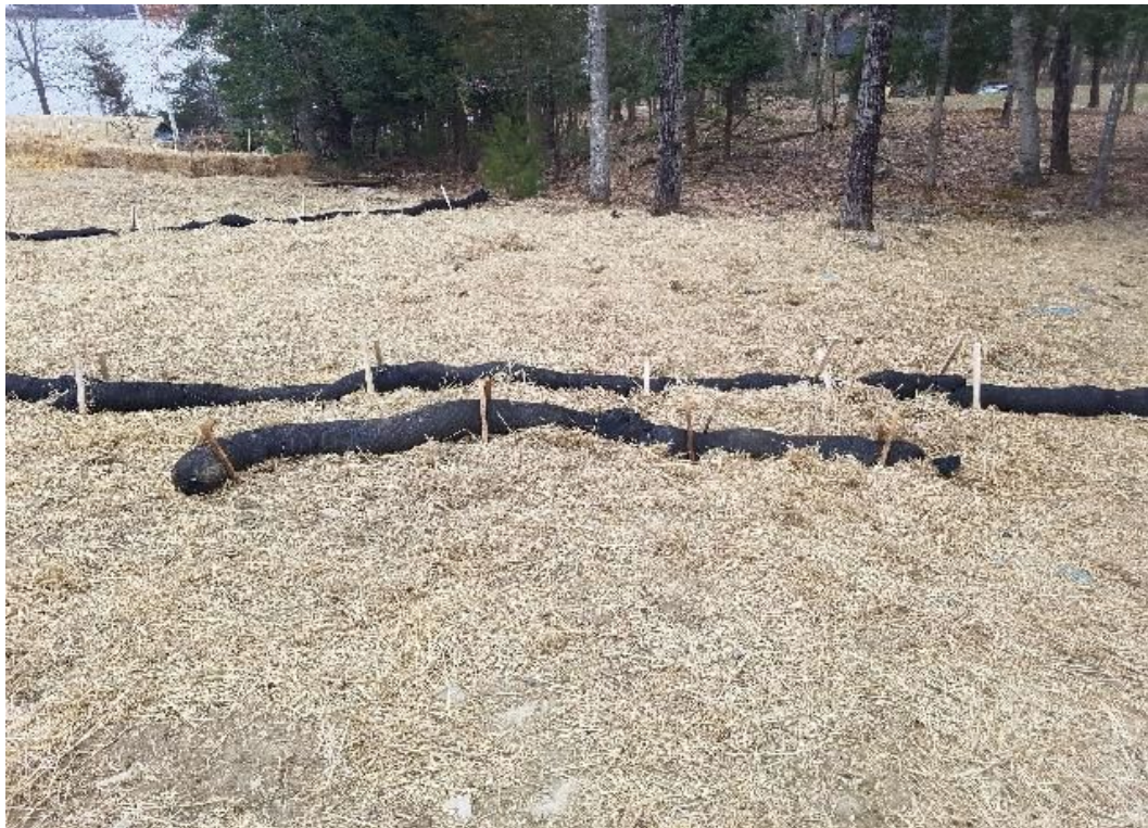
Fig 22: Erosion repaired downslope of Str. 99, filter sock added. Viewing east. (04-01-20).
