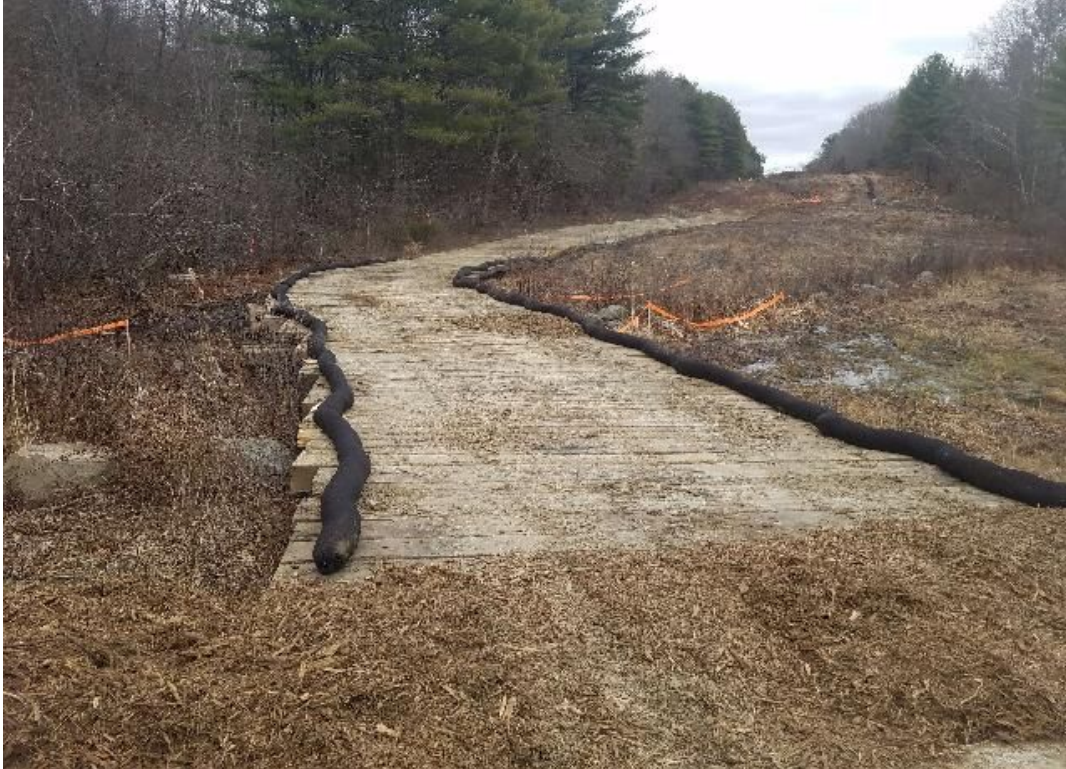
Fig 21: Access road from Str. 85 to 86 through wetland DW 24. Viewing southeast. (04-01-20).
