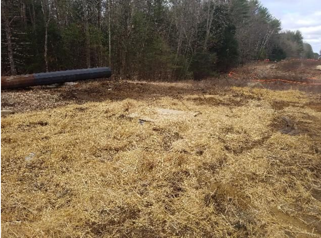
Fig 17: Foundation can set at Str. 77. Viewing west. (04-01-20).
