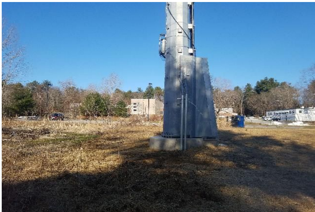
Fig 4: Str. 23 foundation. Viewing west. (03-27-20).
