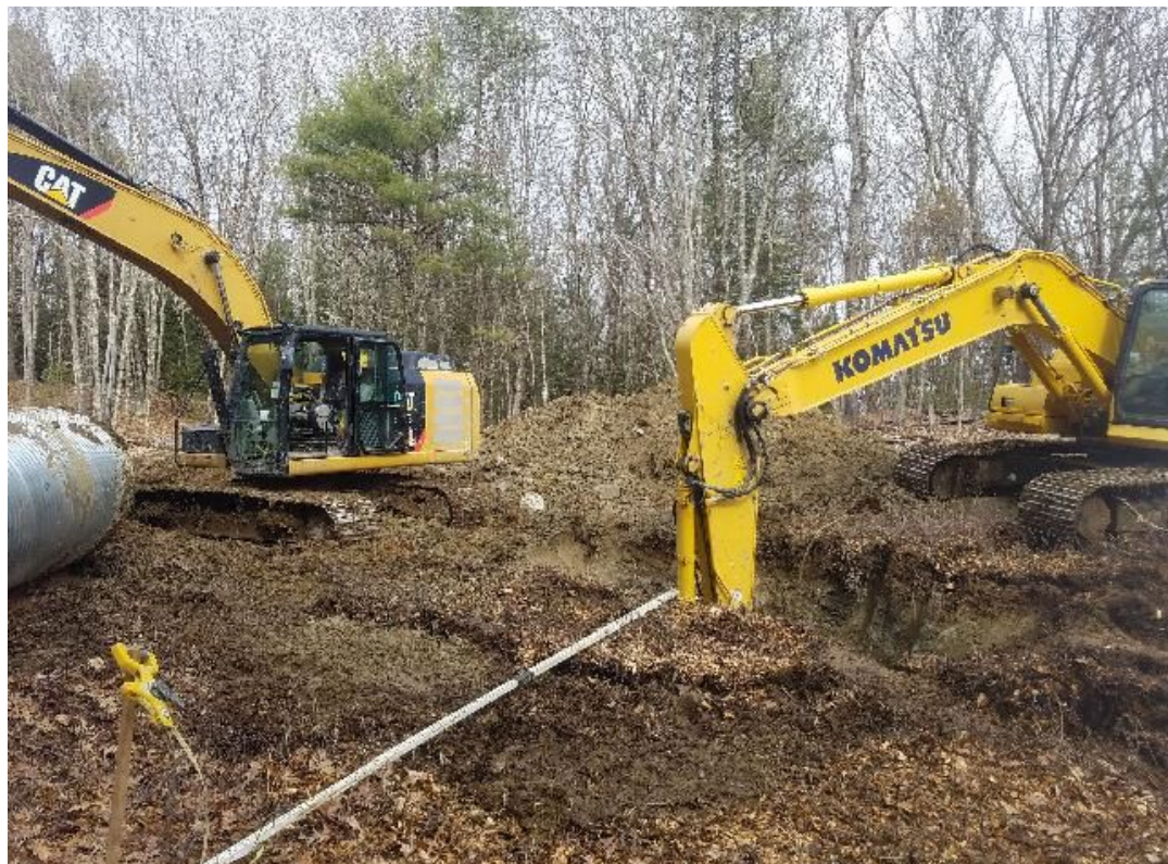
Fig 18: Excavating foundation for Str. 78. Viewing south. (04-01-20).
