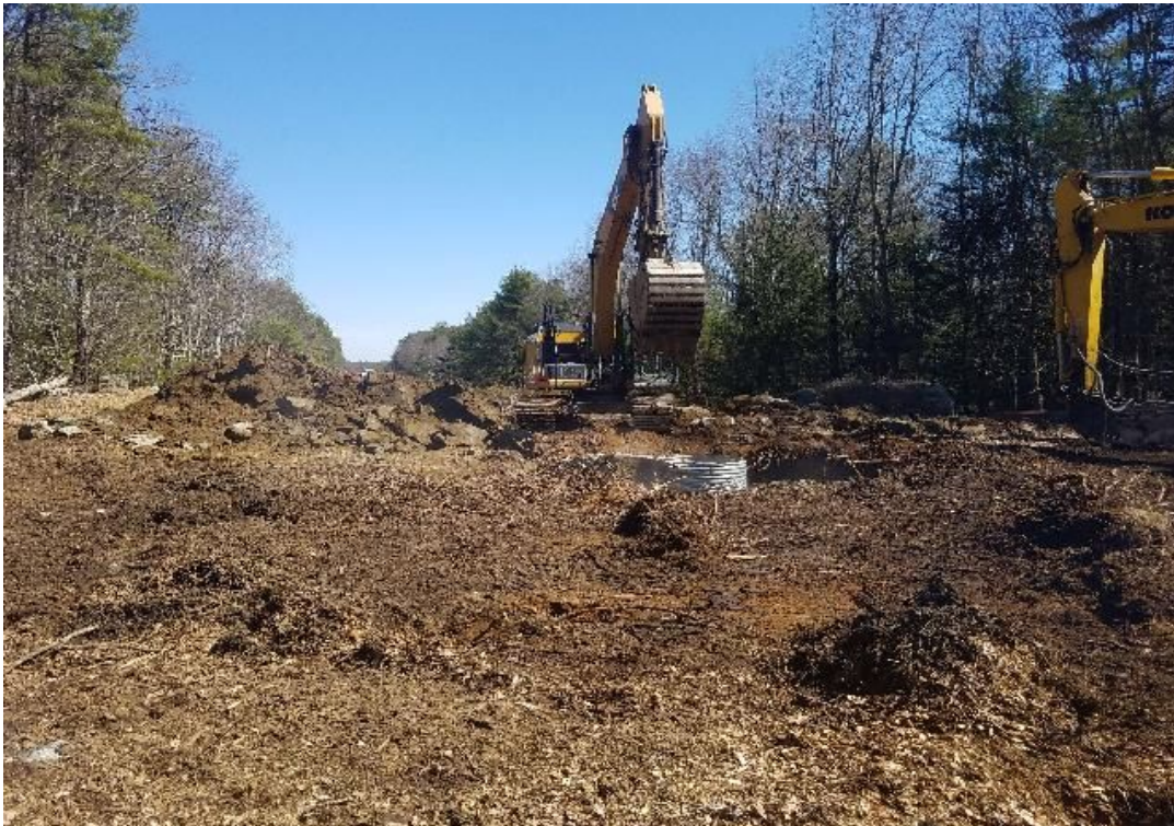
Fig 16: Setting foundation can at Str. 77. Viewing northeast. (03-31-20).
