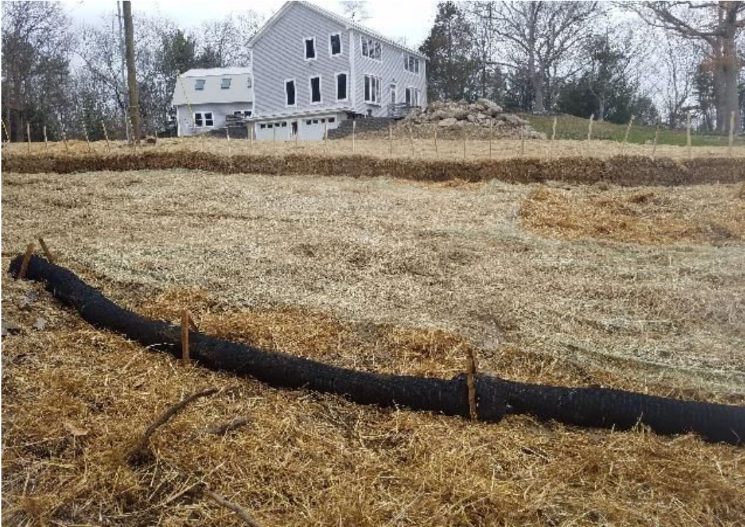
Fig 23: Erosion repaired on slope at Getchell property/west side of the Bay. Viewing north. (04-01-20).
