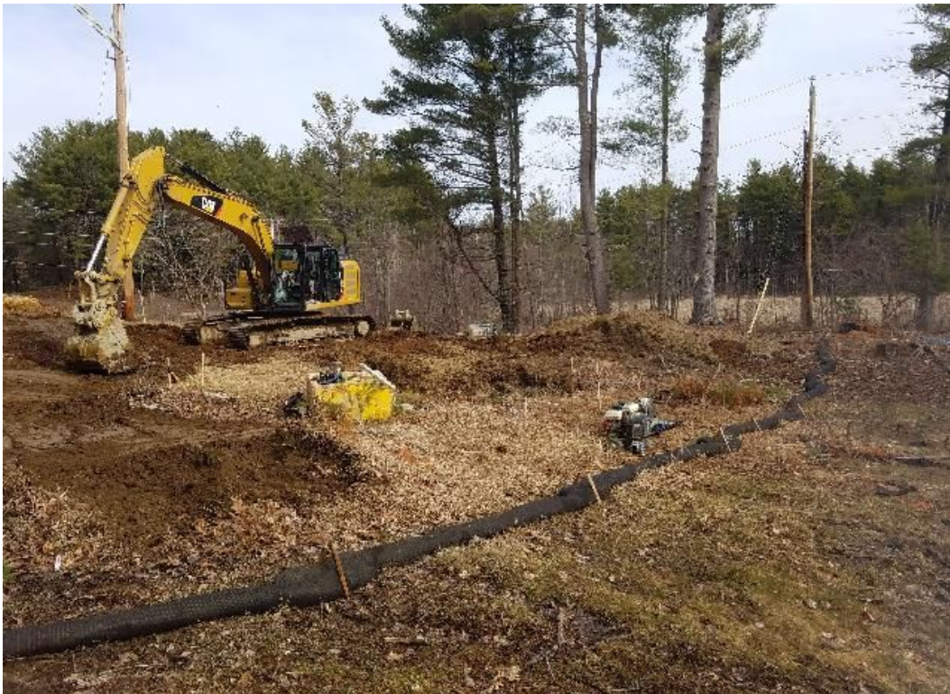
Fig 12: Beginning to excavate foundation for Str. 94. Viewing northwest. (03-31-20).
