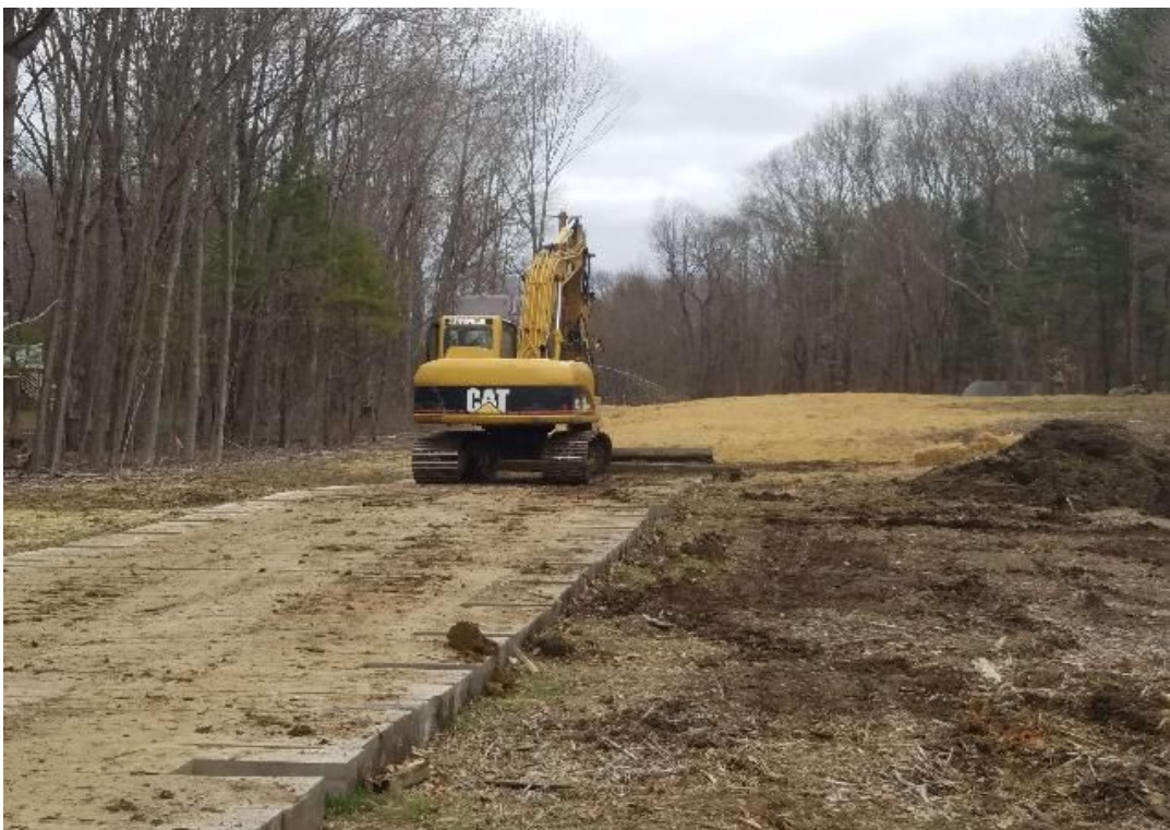
Fig 20: Removing timber mats from access road leading to Str. 107. Viewing northeast. (04-01-20).
