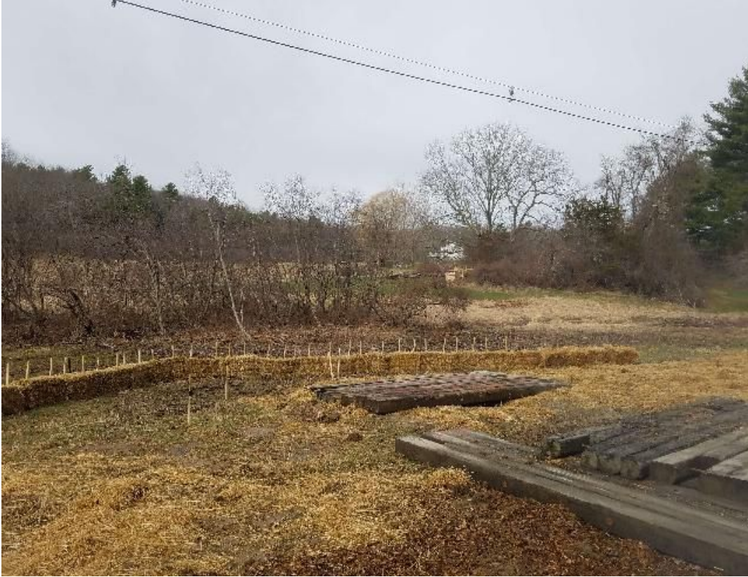
Fig 11: Foundation can set at Str. 95. Viewing west. (03-31-20).
