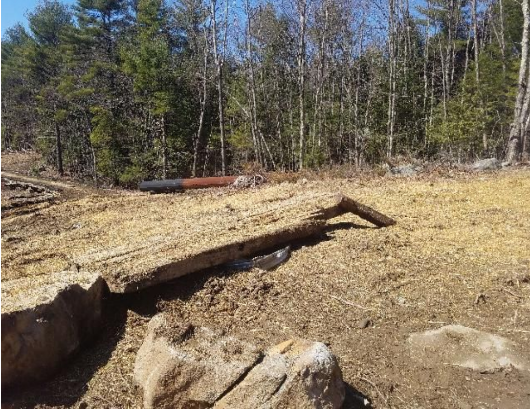
Fig 15: Str. 76 foundation can set. Viewing west. (03-31-20).
