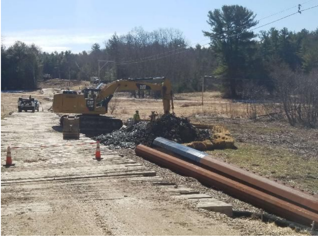
Fig 9: Excavating foundation for Str. 95. Viewing southeast. (03-27-20).
