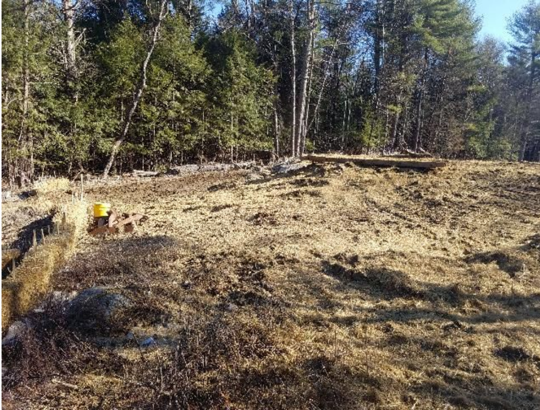
Fig 7: Foundation cans set at Str. 75. Viewing north. (03-27-20).
